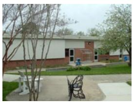
Brick masonry and metal siding
