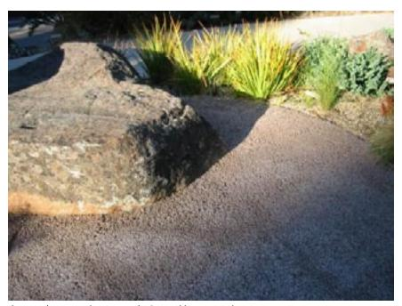
Concrete (porous and non-porous) – Permeable concrete shown
